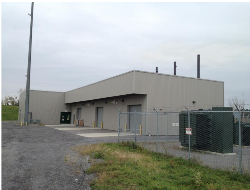
Figure 3: The WCEC gas-to-energy facility
