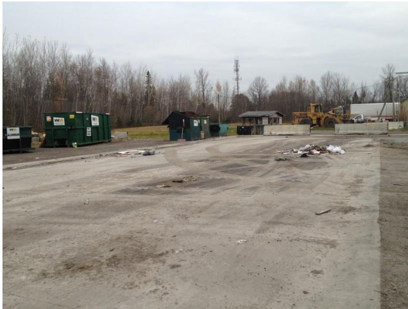
Figure 4: Existing concrete pad at waste transfer facility
